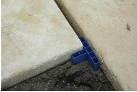
Starting with your first or corner slab, lay the first row of slabs in the direction of the fall. Fit a Gapfast (Cross or Tees as appropriate) paving spacer at each corner ensuring they are placed down in the mortar. Using your hammer/timber tap the slab firmly up against the Gapfasts.
