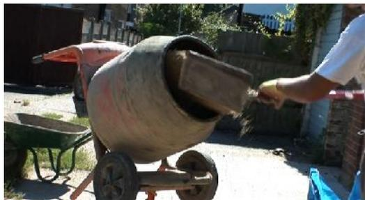
Mix mortar in an electric concrete mixer (again can be hired anywhere) using 6 part sharp sand to 1 part cement, adding just enough water for a stiff-ish mix.
