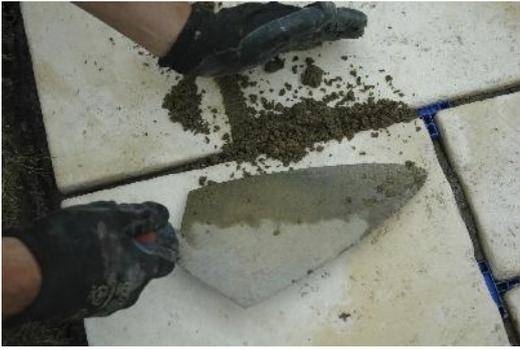
The easiest and quickest way to do this is to fill the joints with kiln dried sand (remember the Gapfasts **paving spacers** stay in the joints) then drench the flags and joints with a suitable Pointing compound (such as Gapfast No-More-Pointing - available early 2013).
