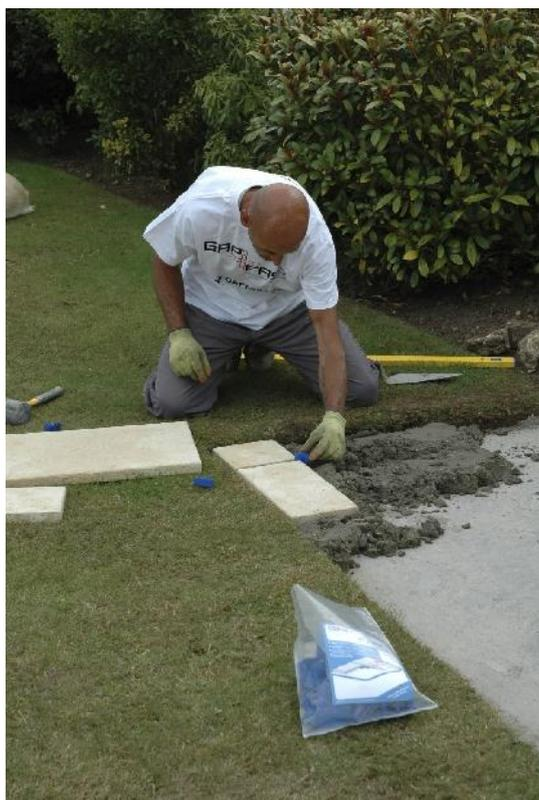
Place mortar to around 50 mm deep onto the prepared base – ‘rippling’ the surface, creating troughs/peaks with a trowel – this will aid tamping / levelling into place.
