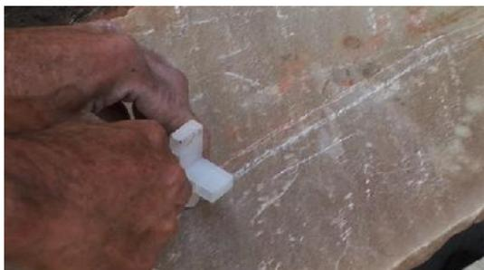
You can also use a Gapfast paving spacer to re-mark your cutting line to ensure you maintain a 10mm joint / pointing gap.
