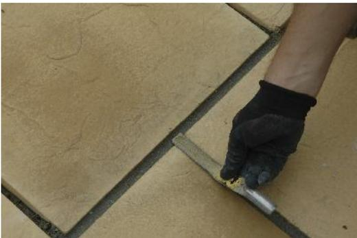
Compact the mortar with a pointing trowel or a piece of wood, and repeat (up to 3 to 4 times) until the joints are full and compacted.
