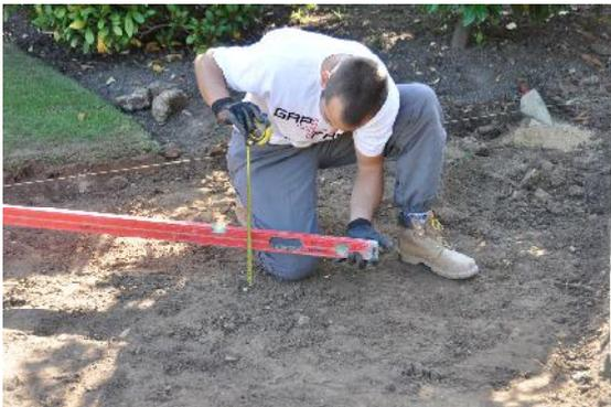
Hammer in wooden pegs to show the finished hardcore level 100 – 120mm above the excavated area, depending on the thickness of your patio slab – allow an adequate fall so rain can run off into the garden. A fall of around 1 in 80 (10 – 15 mm drop in level per meter) is just about right. Then fill up to slightly above the top of the pegs with Type 1 or hardcore; then compact it down, using a vibrating plate compactor (you can hire these almost anywhere).
