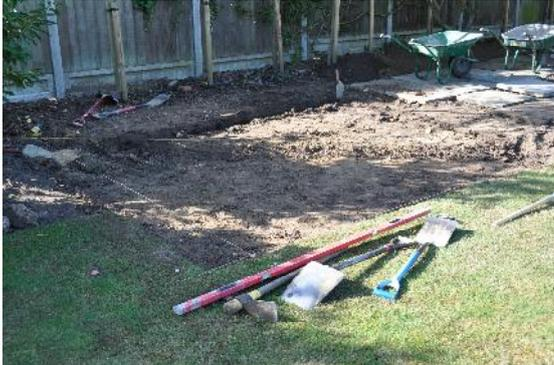
Mark out your new patio using a string line and pegs and check the corners are at right angles, using a builders square.
