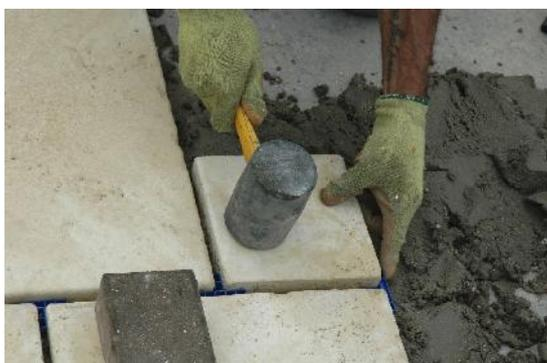
Using a club hammer tap the slab into position. If necessary lift the slab to place a little more mortar underneath. *Note here the Gapfast Tee paving spacer is vertically inserted between the first paving slabs as they are being laid tight against the existing turf border.*
